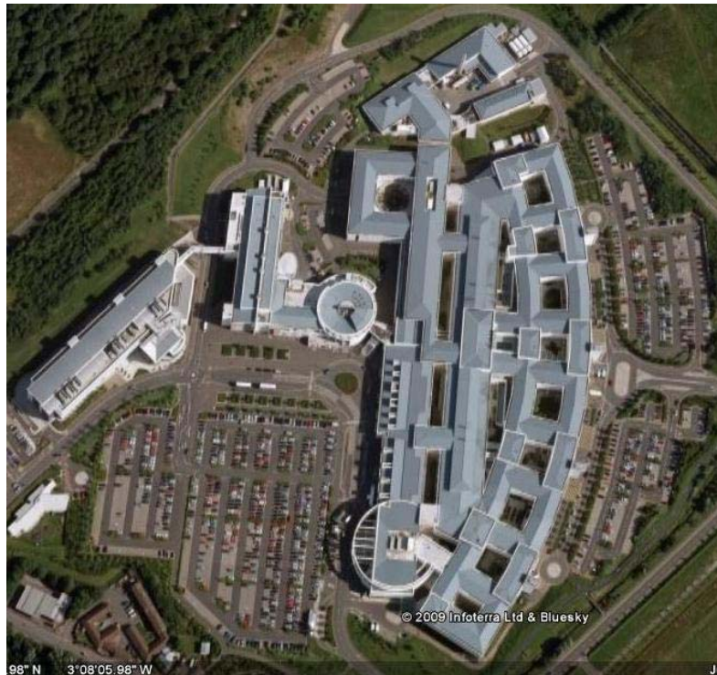
Figure 2 - Aerial view of the Royal Infirmary Edinburgh
