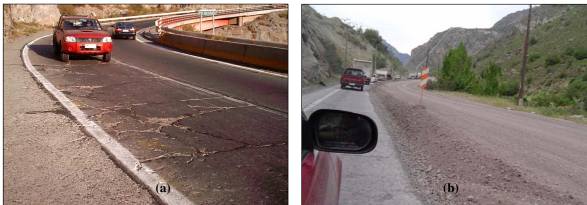
Figure 3: typical pavement original conditions (a) and overlay with granular base (b)
