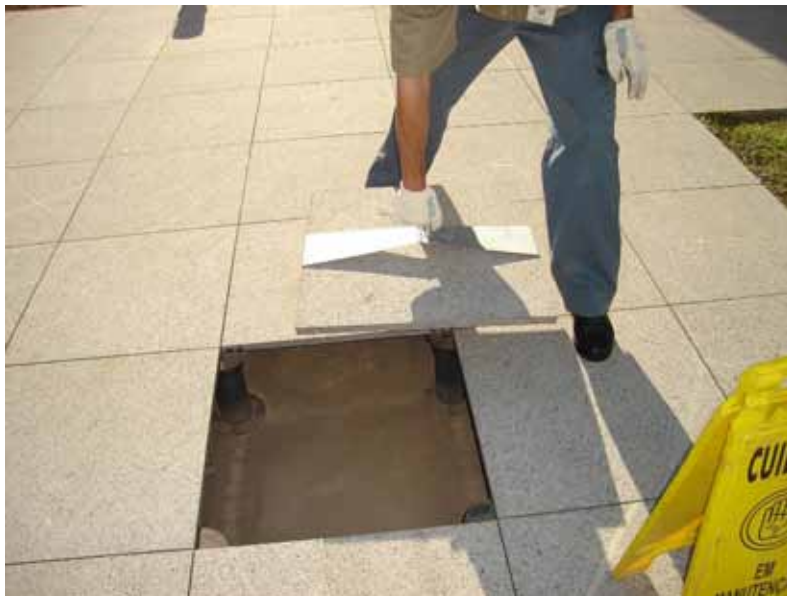
Fig.3 – Simulation of maintenance in a pedestal system with granite slabs in a commercial building in the city of São Paulo (Bernardes, 2009).
