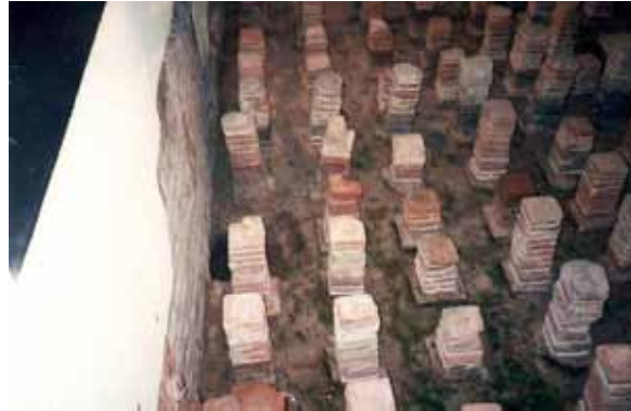
Fig.1 – Ruins of the floor elevated by stacked flagstones from the Roman thermal bath in the city of Bath (Bernardes and Barros, 2009).
