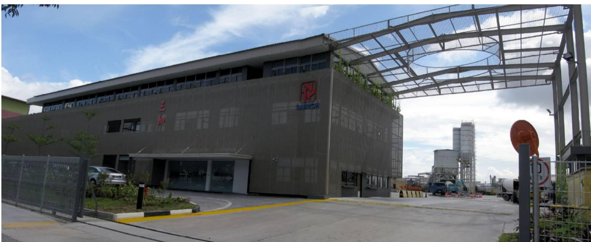
Figure 2: Samwoh Eco-Green Building
