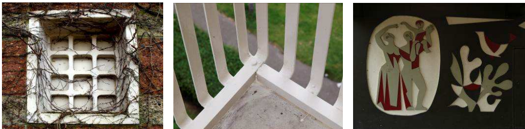
Figure 5. Present day details of exposed concrete and steel in Slotershof Amsterdam.
