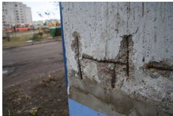
Figure 1. Carbonization (left) and corrosion of the reinforcement of the concrete facade (right).
