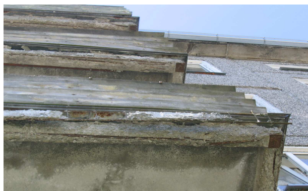
Figure 3. Damages of balcony elements.
