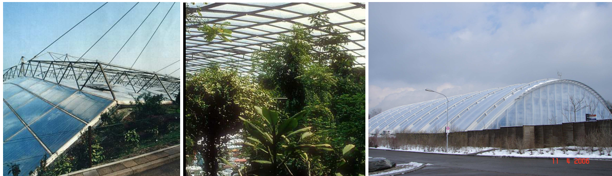
Figure 4, 5 and 6. The roof of bush hall of Burger’s Zoo Arnhem NL (left), inside view (centre) and the Masoala Rain Forest building at Zoo of Zurich (right).
