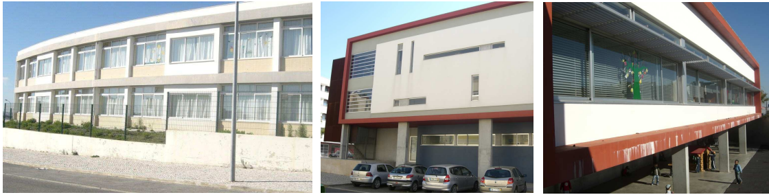
Figure 3. View of school São Bartolomeu (left); Posterior view of Alto da Faia school (centre); South view of Alto da Faia (right).
