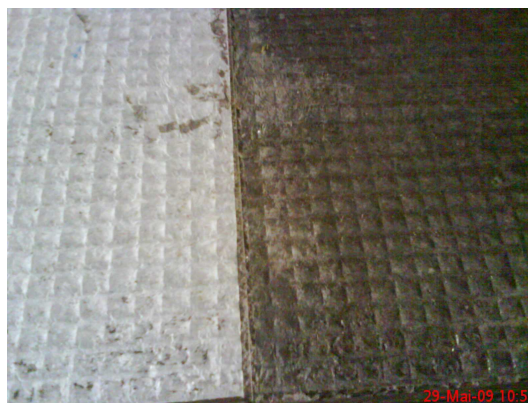
Figure 4. Condition of the mold surface (a) and of the concrete surface after demolding (b).
