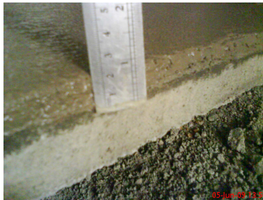
Figure 5. Side view of the grout used during the study.
