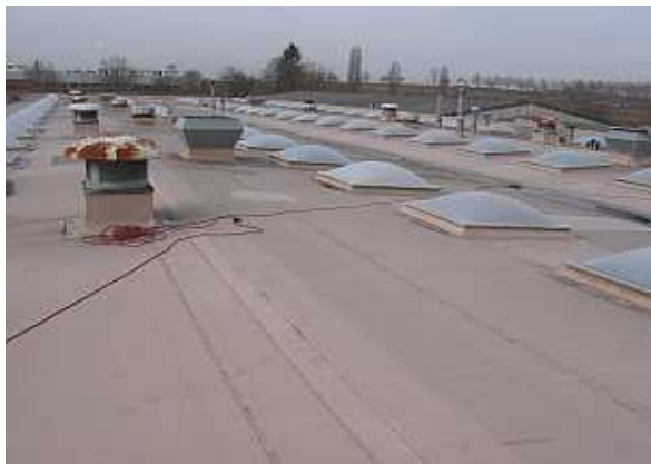
Figure 1. Overview of roof A at Fellbach.
