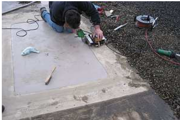
Figure 4. Closing of sampling area on roof C.
