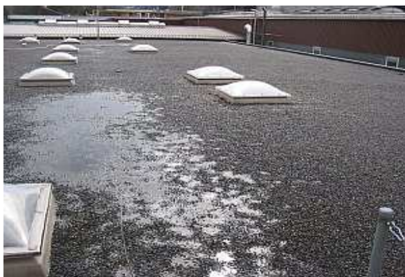
Figure 3. Overview of roof C at Flawil.
