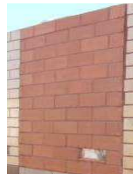
Figure 3. ETICS after 2 years of weathering (with 80 mm standard joints).
