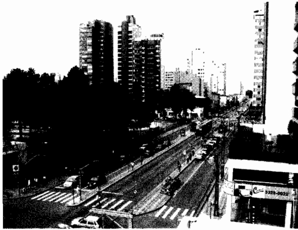
Fig. 3 – Image of the Southern Structural Axis in Curitiba, Sete de Setembro Avenue, in 2008 (DZIURA, 2009)
