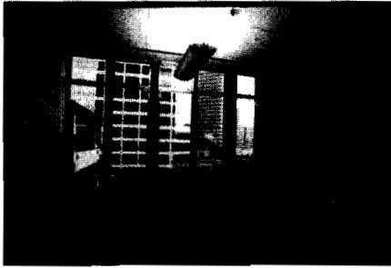
Figure (16) Before direct sunlight enters the windows, The electrochromic windows are in the clear state.
