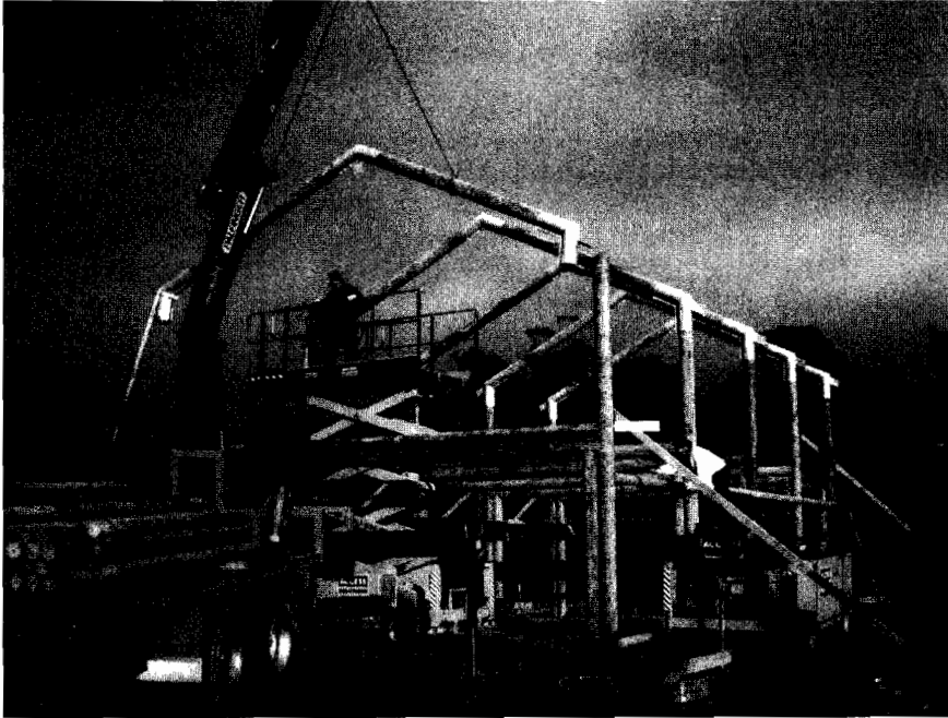
Figure 11: UDR portal structure for 2 storied building
