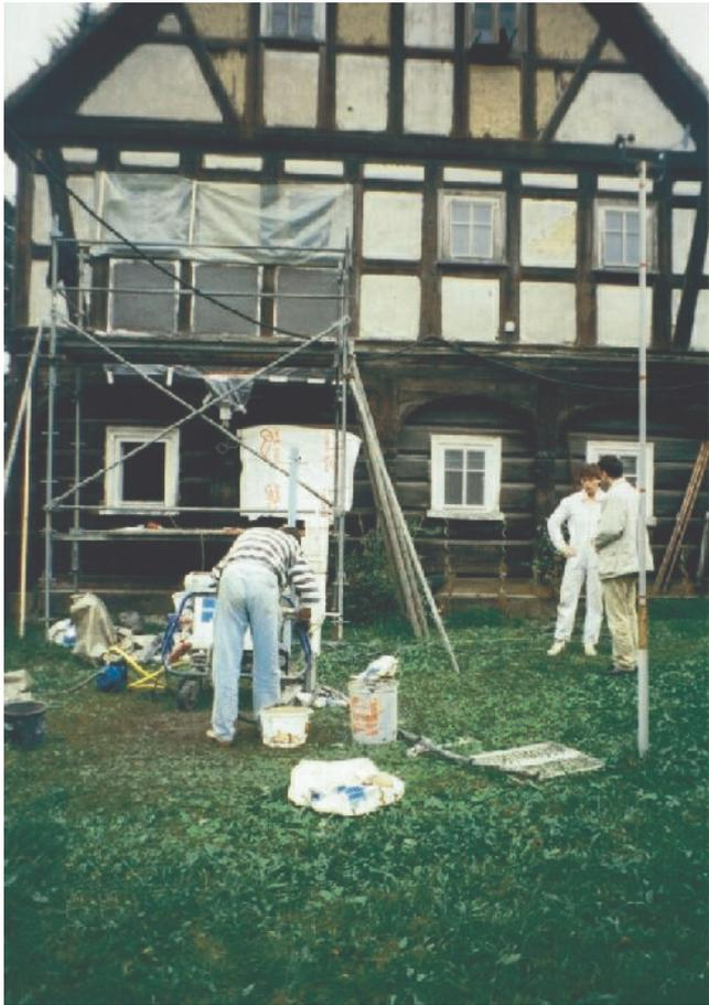
Fig. 12. Installation of the new framework filling in the test building in East Saxony.
