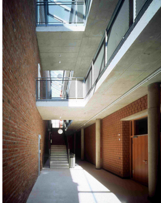
Figure 7 View inside the atrium, it shows the open thermal masses and the internal clay wall used for all the installations (right hand side) (Meyer 2001)
