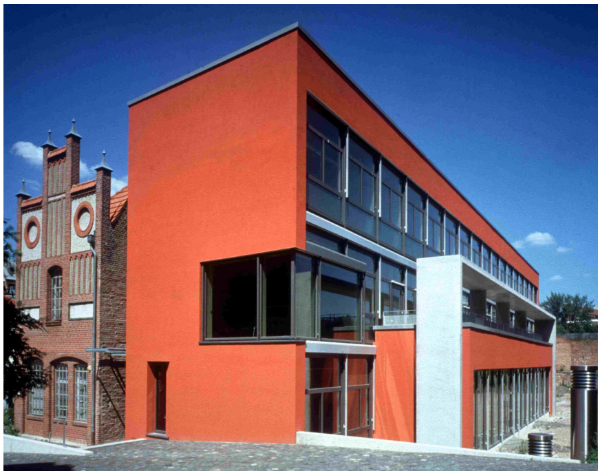
Figure 1 The office building of the Centre for Sustainable Building (Meyer 2001)
