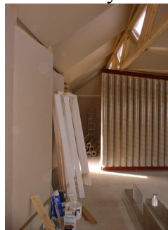
Figure 5: Tube wall in place
