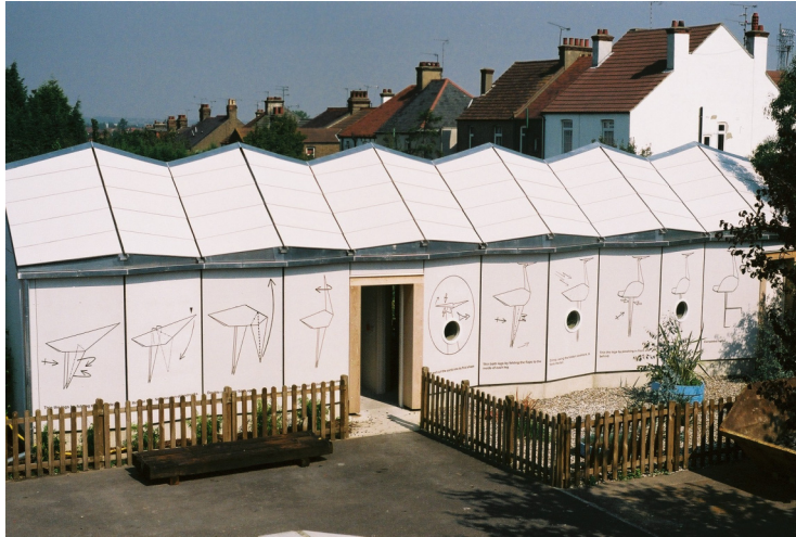
Figure 8: The finished building
