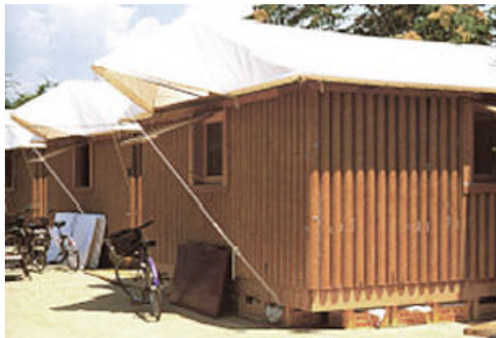
Figure 1. Paper tube houses for the Kobe earth quake victims
