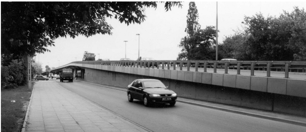
Fig. 3 Viaduct on Hynka street in Warsaw –supervised by ITB (Concrete Department).
