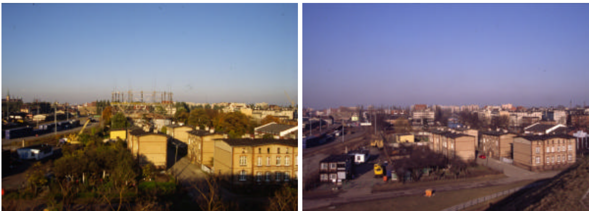
Figure 3. Gdansk, site of former gas plant before and after dismantling of the riveted iron gas tank
