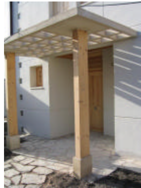
Picture 2.South facade and atrium
