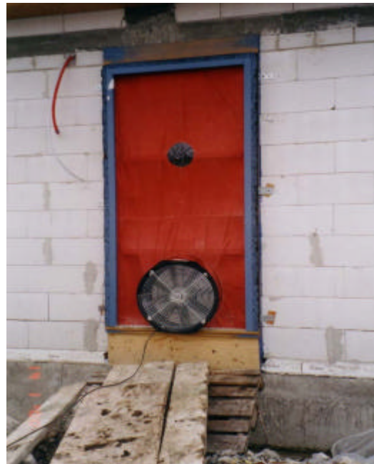
Figure 4. The blower in the door during the test
