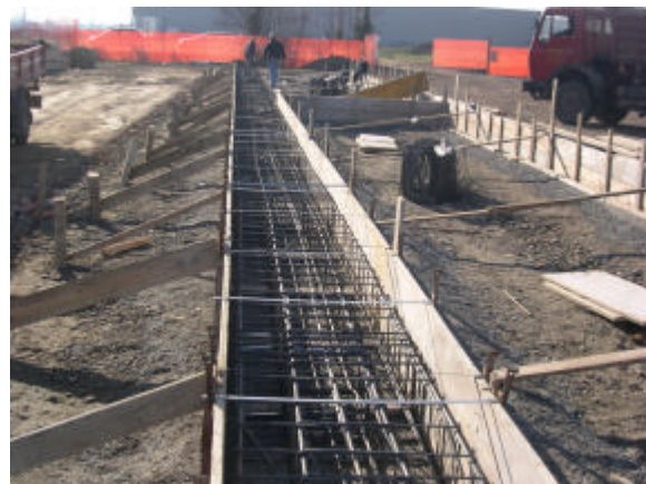
Photo 2. Preparing the foundations
