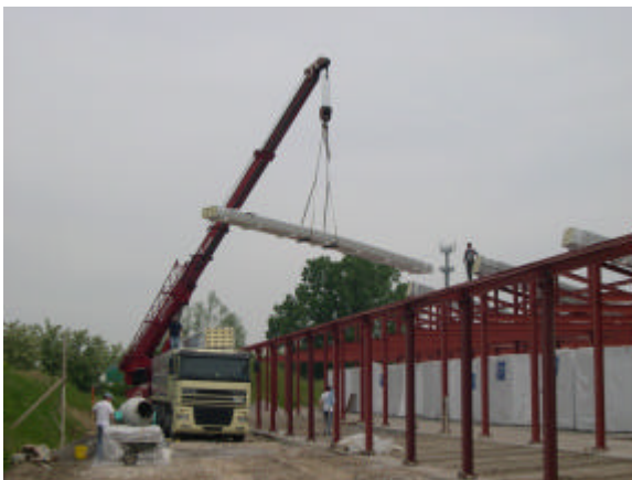
Photo 1. Assembling the roof
