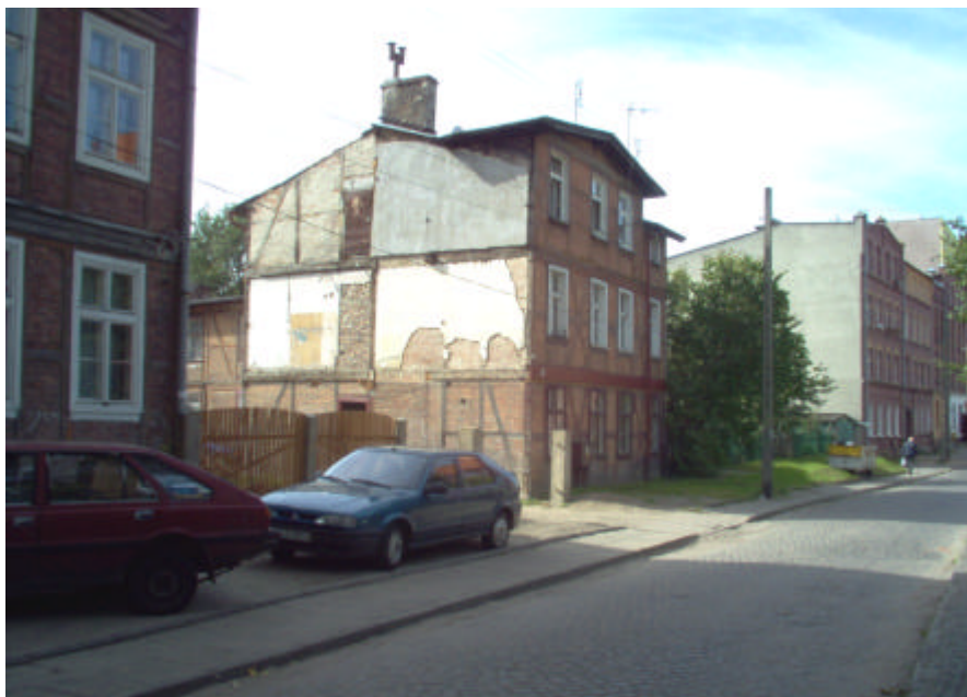
Photo 1. Gdansk, Malczewskiego Street, not-used land after demolition works
