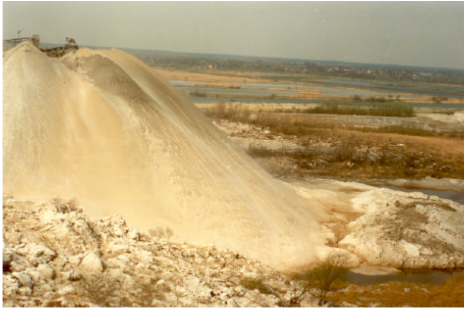
Fig. 6. Damping site of phosphor-gypsum Police near Szczecin 40 m high. Deposited -3 mln cubic meters of chemicals.
