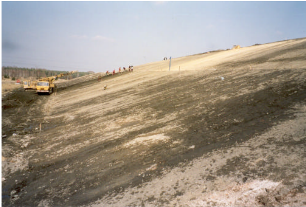
Fig. 8 Post-operational land reclamation of chemical plant in Tarnowskie Góry . (recultivated ground surface ca. 70 ha, 4 landfills ca. 2 millions m 3 of waste).
