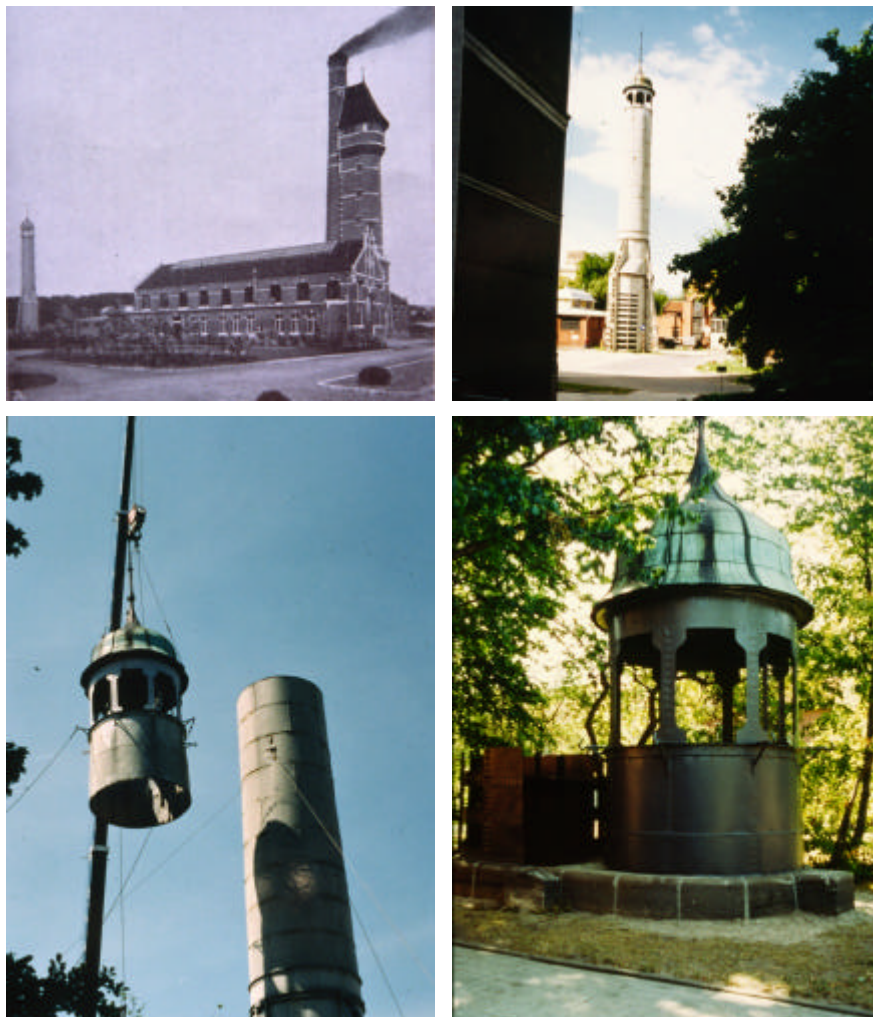
Figure 4. Gdansk University of Technology; relocation of the iron cooling tower (1902-1994) (photo T. Chmielowiec).
