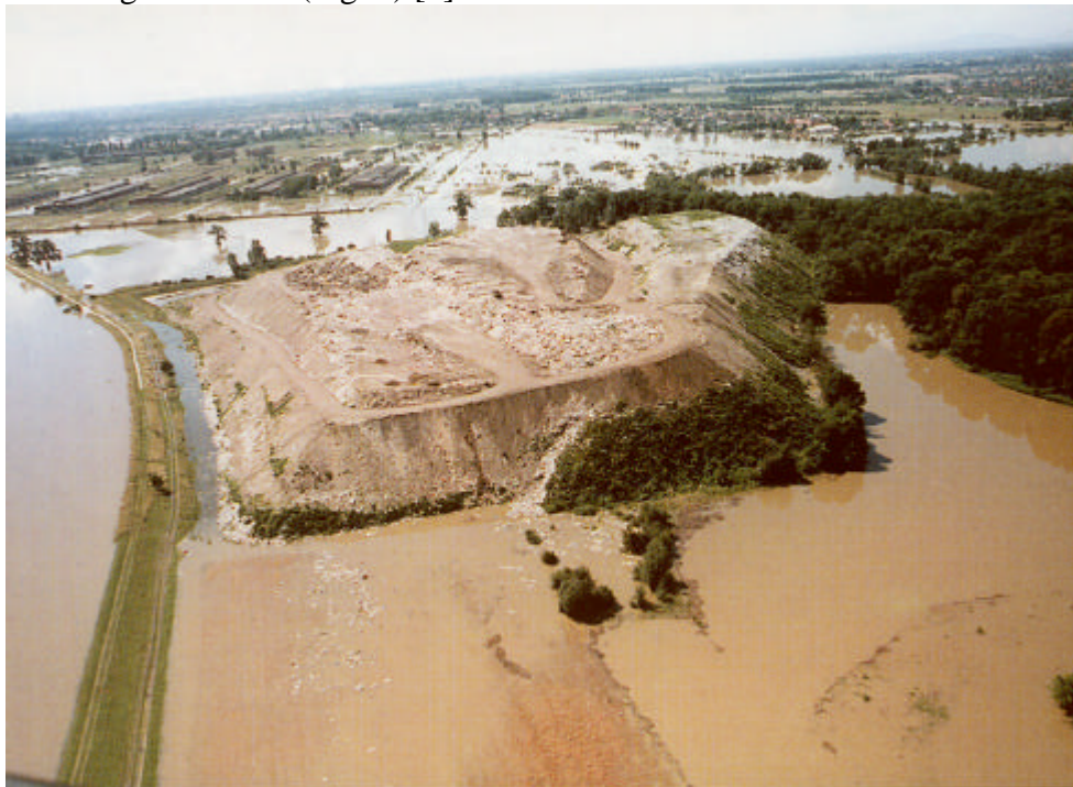
Fig.7 Waste fills near Wrocław during the flood in 1997
