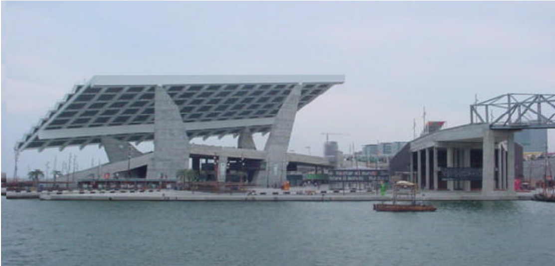
Figure 1. Photo-voltaic pergola at Barcelona’s Universal Forum of Cultures produces 1.3 megawatts of electricity; “roughly the consumption of 1,000 Spanish homes” [8]. Metamorphosis of the technical solution into an art form and an exemplar of the enduring temptation to customise built artifacts around new technologies [9]
