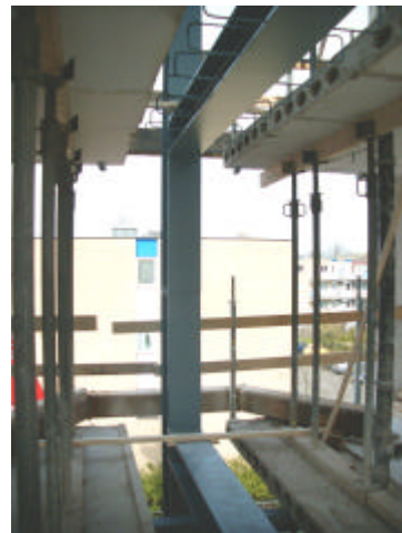
Figure 5. Situation after installation of the steel frame
