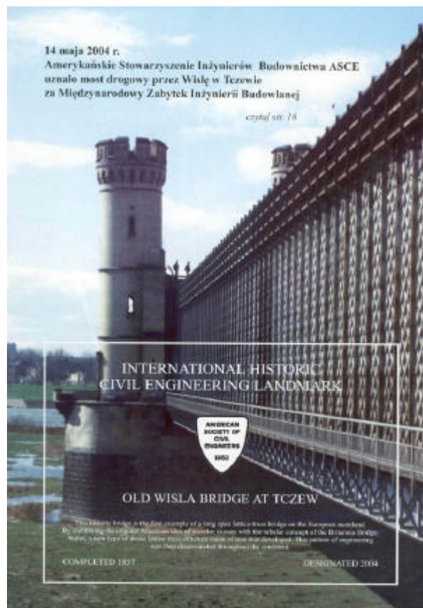
Figure 5. Tczew, road bridge over the Vistula river after repair as shown on the cover of the Gdansk UT Newsletter "Pismo PG", No. 6 (100) 2004 (photo: W. Affelt).
