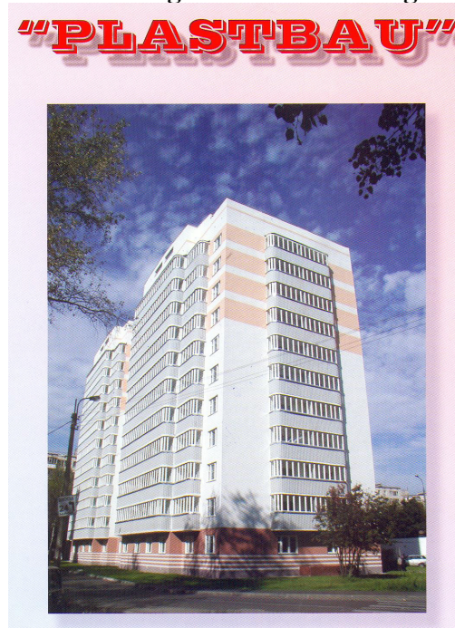
Figure 4. The residential building for the monitoring of energy performance
