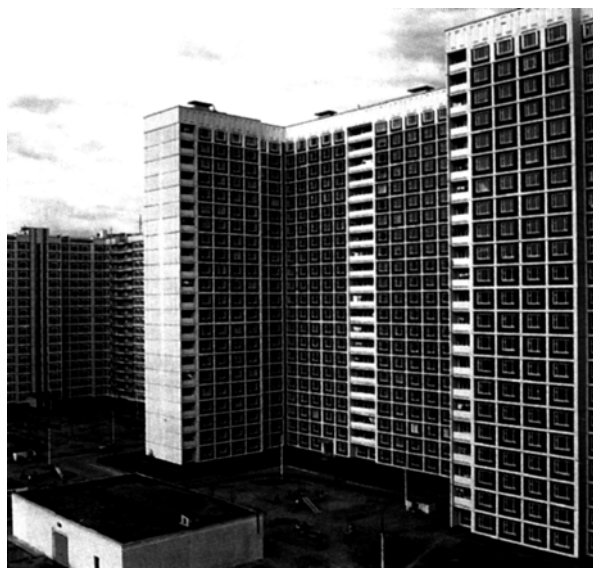
Figure 2. Visually negative inexpressive house
