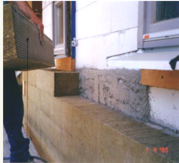
Figure 2: Insulation with mineral wool, 30 cm thick
