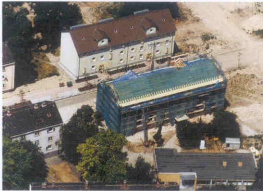
3. The 3-Liter House under construction.
