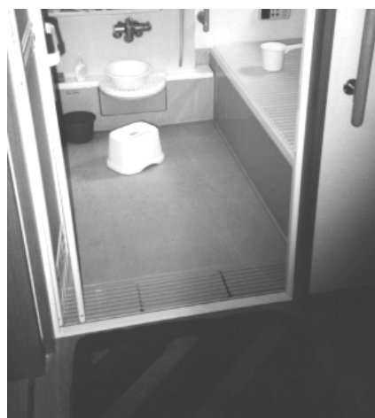
Photo 6. Entrance to the bathroom is flat.
