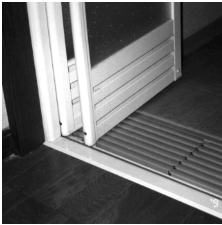
Photo 7. Close-up of flat doorsill.
