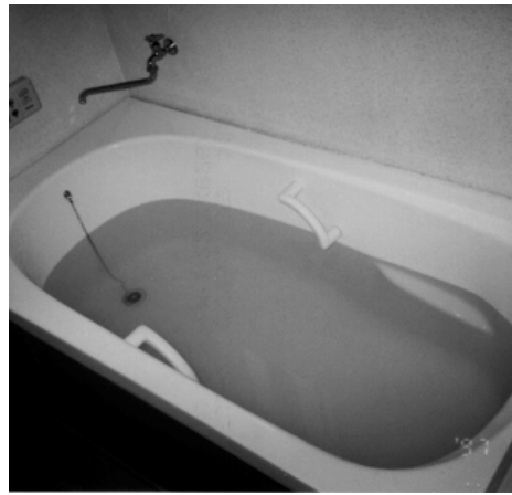
Photo 8. Bathtub with grab bars.
