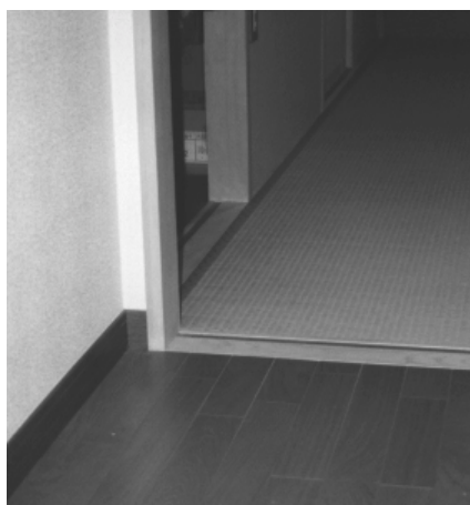
Photo 3. Floors are basically without raised door sills.
