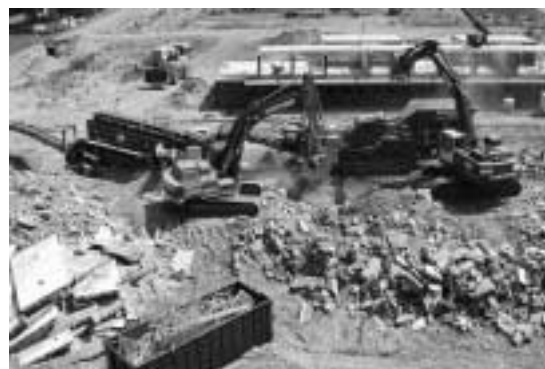
Fig 2: Mobile crusher on demolition site
