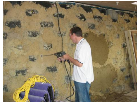
Figure 2 Tyre wall undergoing sensor installation
