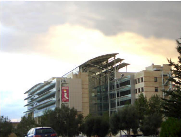
Figure 6 Electricity Authority of Cyprus Headquarters, Nicosia, Cyprus
