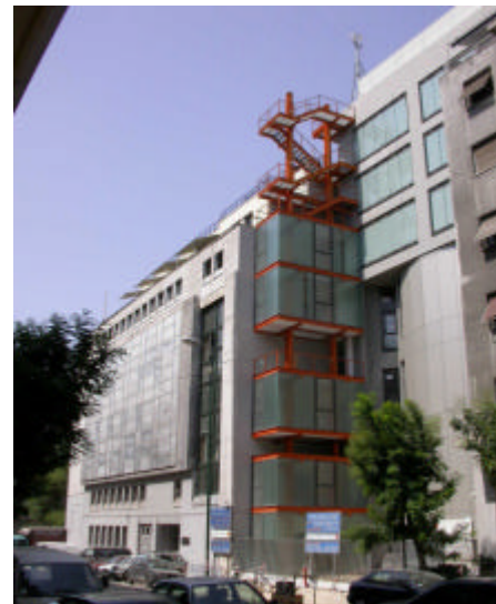
Figure 3 Power Distribution Centre, Athens, Greece
