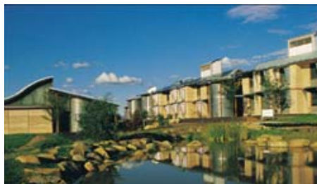
Fig. 1.2a: School of Environment and Information Services. Charles Sturt University Thurgoona Campus. http://www.csu.edu.au
