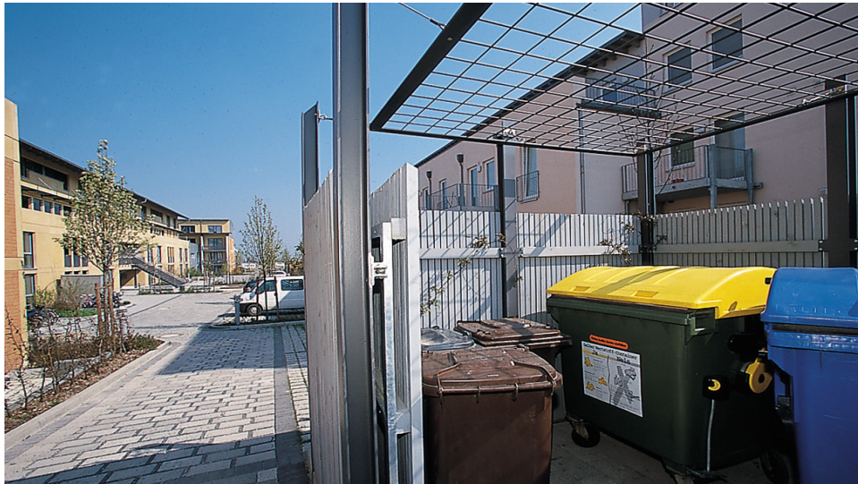
Figure 4 Waste collection point
