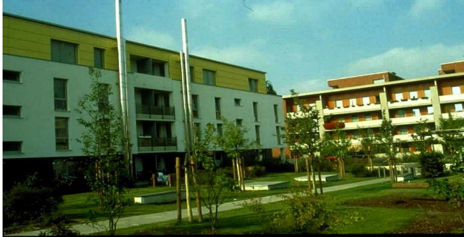
Figure 2 Decentral cogeneration plant in residential block basement
