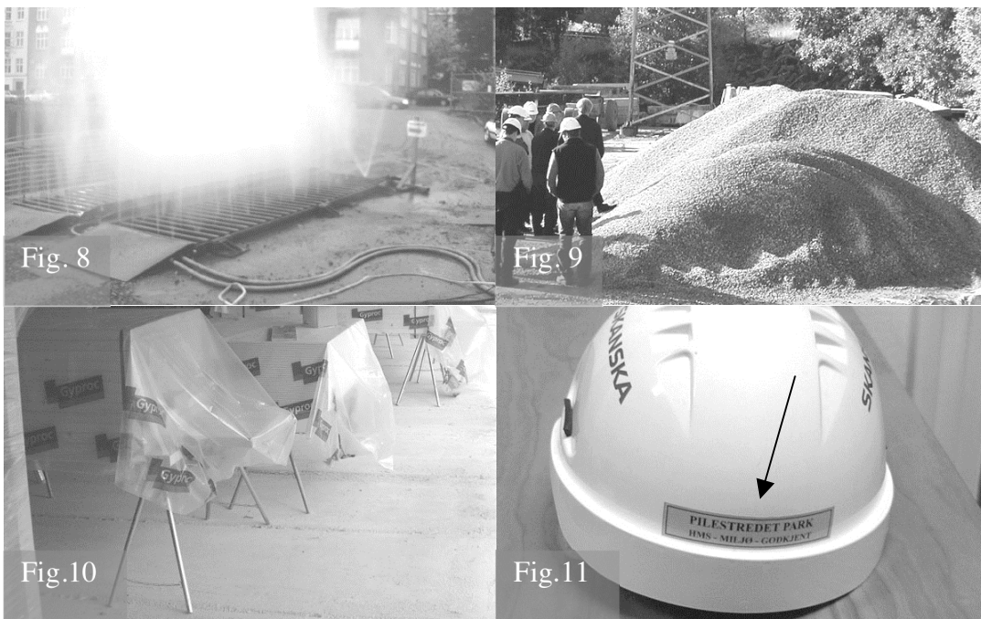
Fig. 8: On-site vehicle wheel cleaner. Fig. 9: Grinded wasteproducts for reuse in concrete slabs. Fig. 10: elevated board stacks for easy floor cleaning and reduced manual lifting height. Fig. 11: Helmet sticker certifying for on-site work after receiving information on environmental programme.
