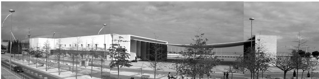
Figure 1 - Eastern view of the Portuguese Pavilion Building, with the suspended concrete canopy.
