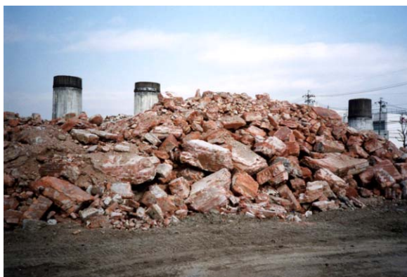
Flue dismantling created enormous quantities of bricks
