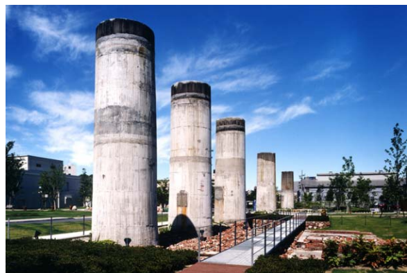
Smokestacks and flue
