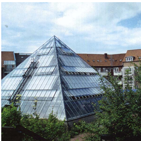
Figure 3 not well working Living Machine, Kolding
