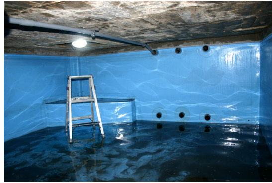
(b) After refurbishment
