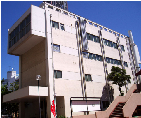
(a) Before refurbishment
