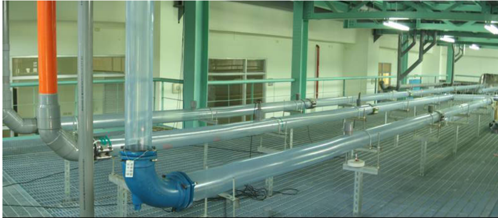
Figure 2 the pictures of main drain testing rig
