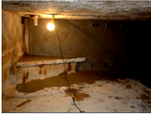
(a) Before refurbishment
