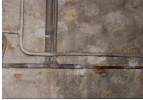
Figure 4 – Lead pipe in a house system
