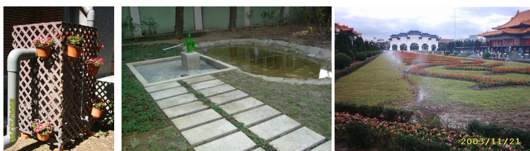
Figure 3- Installation of rainwater reuse irrigation facilities
