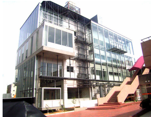
(b) After refurbishment
