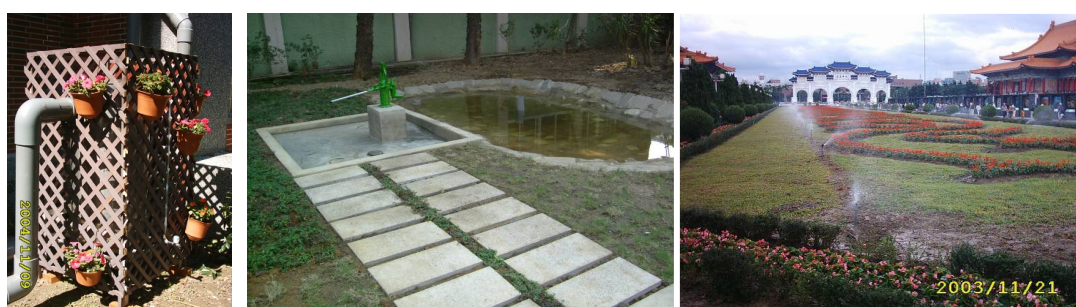
Figure 3- Installation of rainwater reuse irrigation facilities
