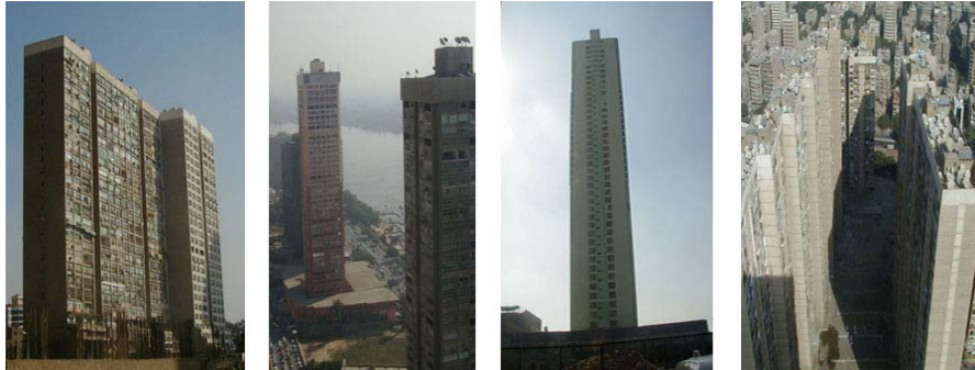
Figure 6.1 High-rise example from Egypt
