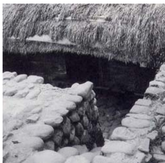
CIB2007-344 Figure 1.7 Stone foundation CIB2007-344 Figure 1.8 Covered cogon-grasses
