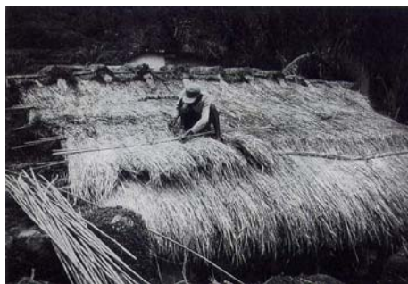
CIB2007-344 Figure 1.7 Stone foundation CIB2007-344 Figure 1.8 Covered cogon-grasses
