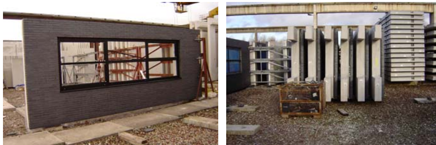
Figure 3 Mounting of casings and glazing; storage of the units
