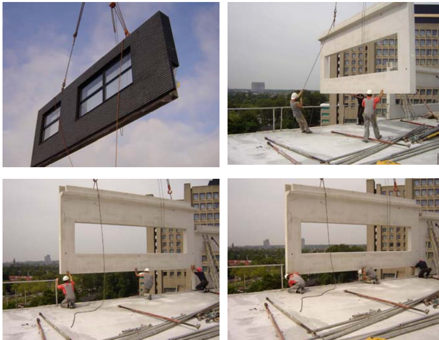
Figure 4 Getting the façade unit in the right position
