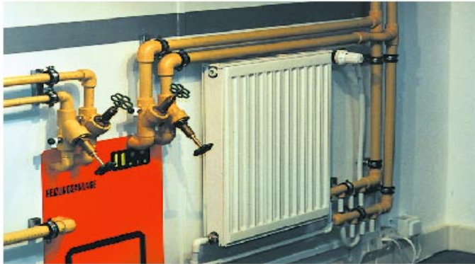
Figure 8 – PP-R systems for radiator connections
