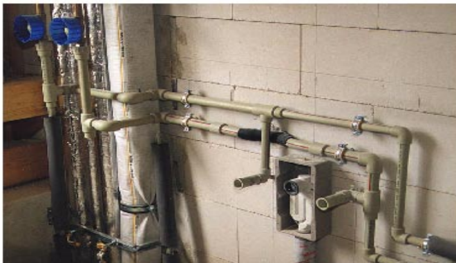
Figure 6 – PP-R drinking water installation
