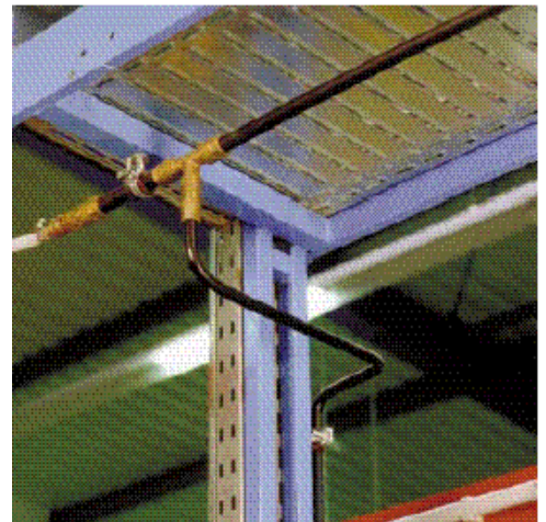
Figure 6 – PP-R drinking water installation
