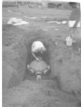
Figure 7: Installation of Radial Plastic Inspection Chamber
