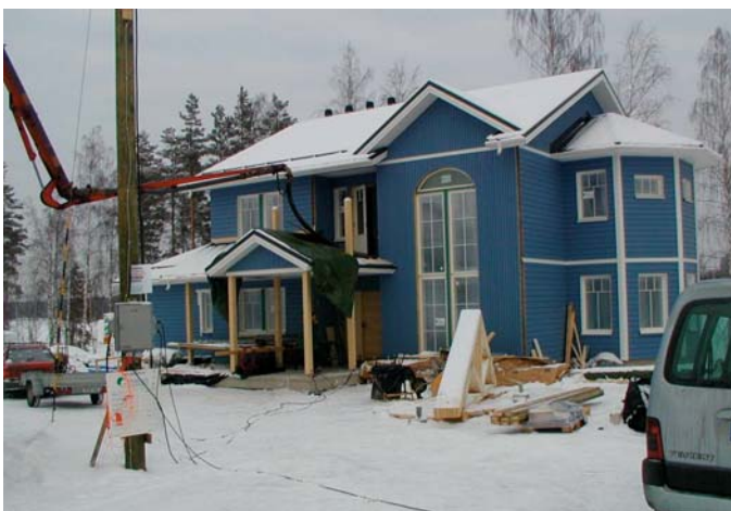
Fig. 2. Construction site in February 2003
