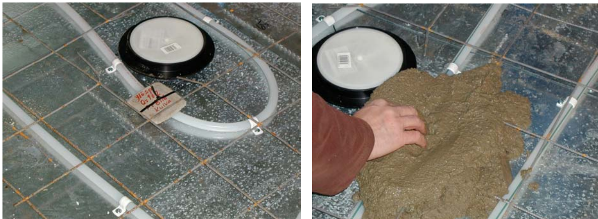
Fig. 3. Pre-cast sensor before casting intermediate floor slab
