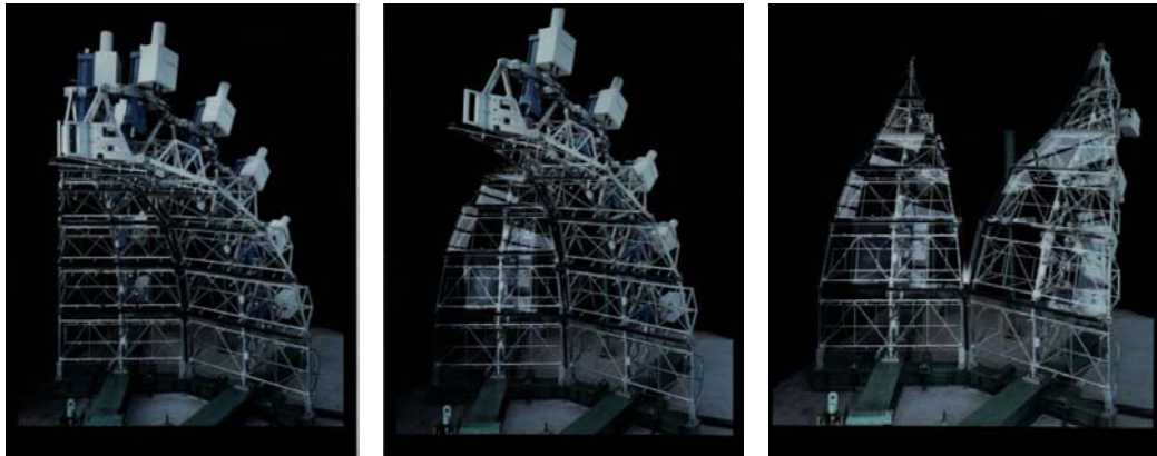
(1) Completed Closing (2) One of Roof was Closing (3) Moving Roofs to Several Shape and the Other was Opening
