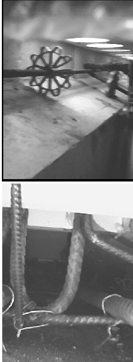
Figure 9: photo's inside a foundation beam (after refilling soil and before pouring mortar). Above: part of top flange of I-shaped beam. Below: part of bottom flange.
