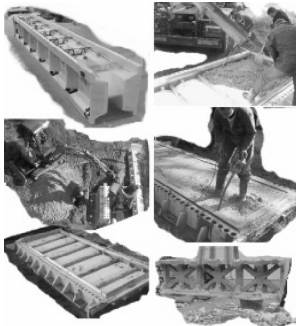
Figure 12: impression of pilot project. left-top: prefab form with reinforcement before applying edge form; left-middle: excavator prepares, levels, digs, shifts, positions and refills; left-bottom: ground floor and formwork ready for concrete; right-top: pouring of concrete (foundation + ground floor); right-middle: compacting; right-bottom: dismantled foundation.
