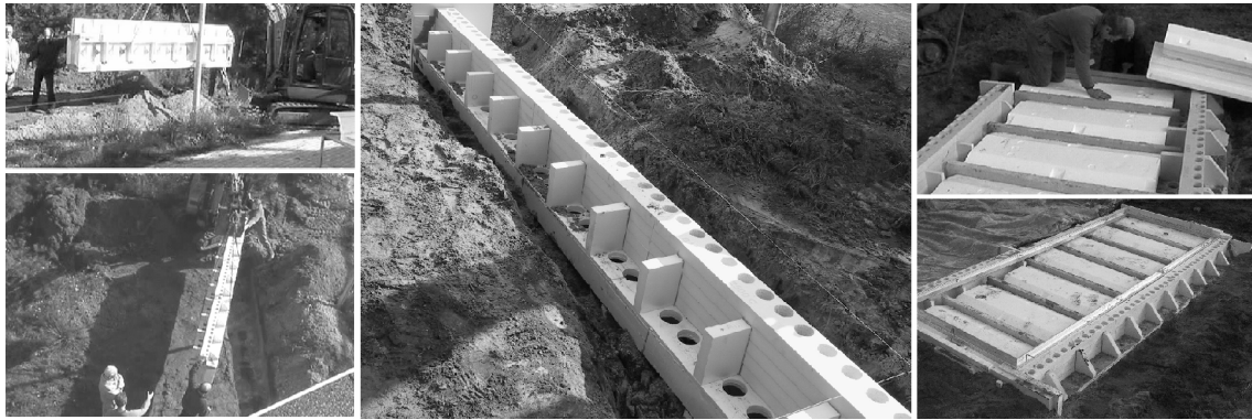
Figure 8: Left: the excavator is used to put in the prefabricated formwork. Middle: Formwork with refilled soil. Right: Next the ground floor is prepared, here a PS-combination type is used.
