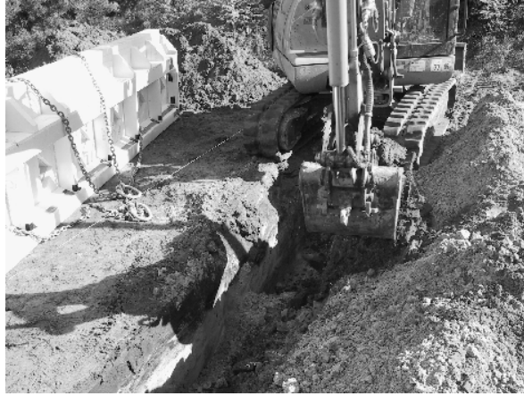
Figure 7: The excavator makes trenches, puts formwork in and refills in running actions.
