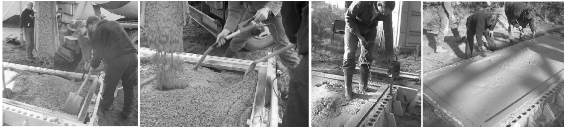
Figure 10: Left: Mortar is poured on top of the floor. Middle: Mortar flows into the foundation with openings that make compaction possible. Right: Finished floor and foundation.
