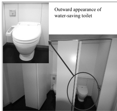
Photograph 1 Outward appearance of fourth floor men's restroom
