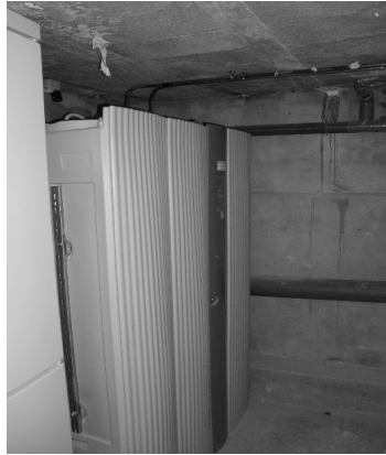
Figure 3 – Water treatment system
