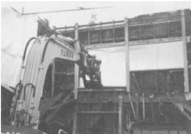
Photo 1 Deconstruction site of the post and beam wooden house.
