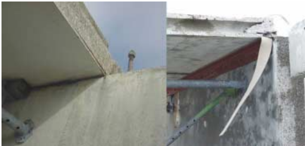
Figure 7: The situation after dismantling and the solution.
