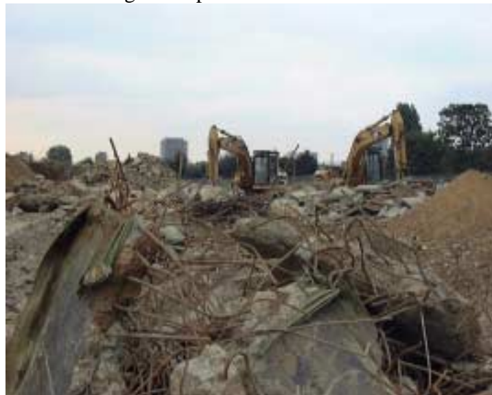
Crushing and separation of demolition waste
