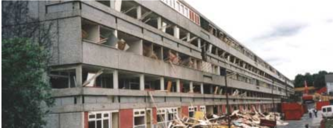
Photo 2. Materials stripped from flats are left on access decks for sorting.
