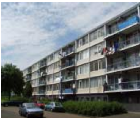
Figure 4: Old apartment building
