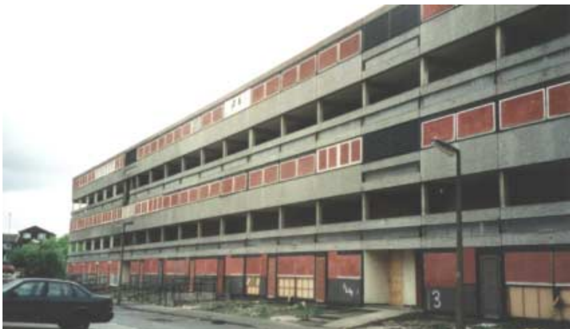
Photo 1. A section of the north elevation of Jespersen Street before demolition.
