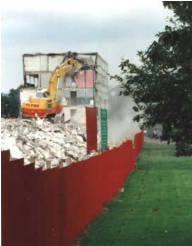
Photo 3. The 75 tonne excavator gains the height it needs using the debris pile.
