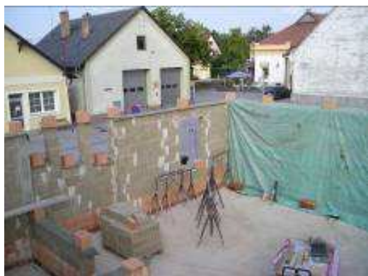
Fig. 3 Durable water protection during execution
