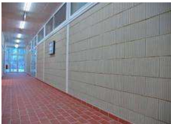
Fig. 1 Unfired loam brick before optimisation, used not load bearing Fig. 2 First prototype of optimised unfired loam brick
