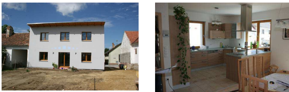
Fig. 8 Finished LEHM.konkret pilot building project
