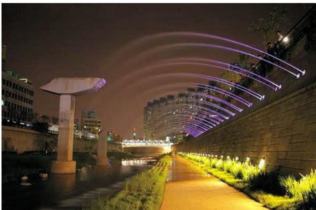
Fig.10. Night view of the tunnel-waterfall with the existed bridge piers of elevated road structures
