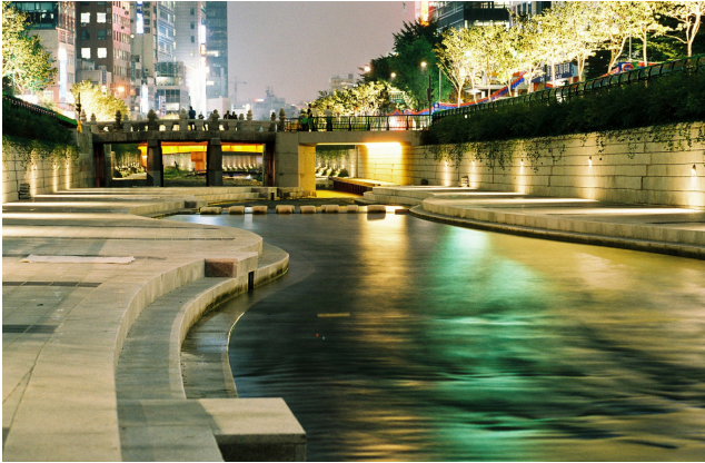
Fig.9. Night view of the restored historical Gwangtong Bridge
