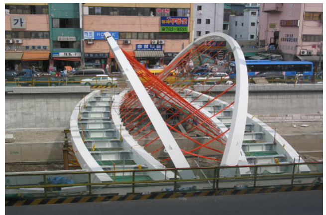
Fig.8. A pedestrian bridge under construction
