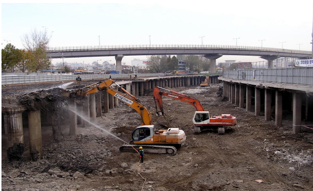
Fig.4. Dismantling the elevated roads (top) and the covered structures (bottom)
