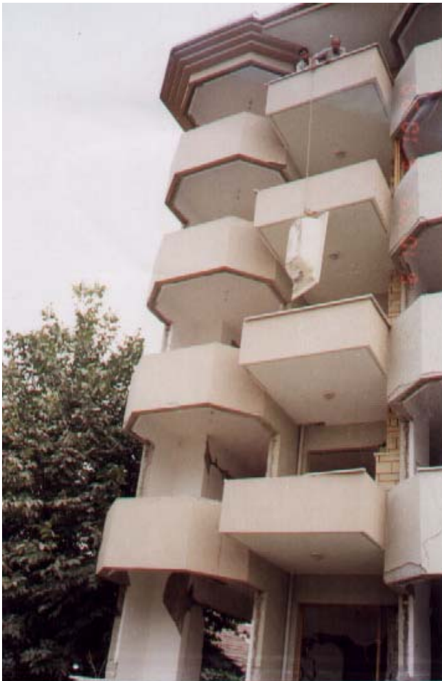
Figure 14: Deconstructing a severely damaged, newly constructed building in Golcuk: Bath tub being lowered from the 5th floor of the building whose ground floor had buckled under [i].
