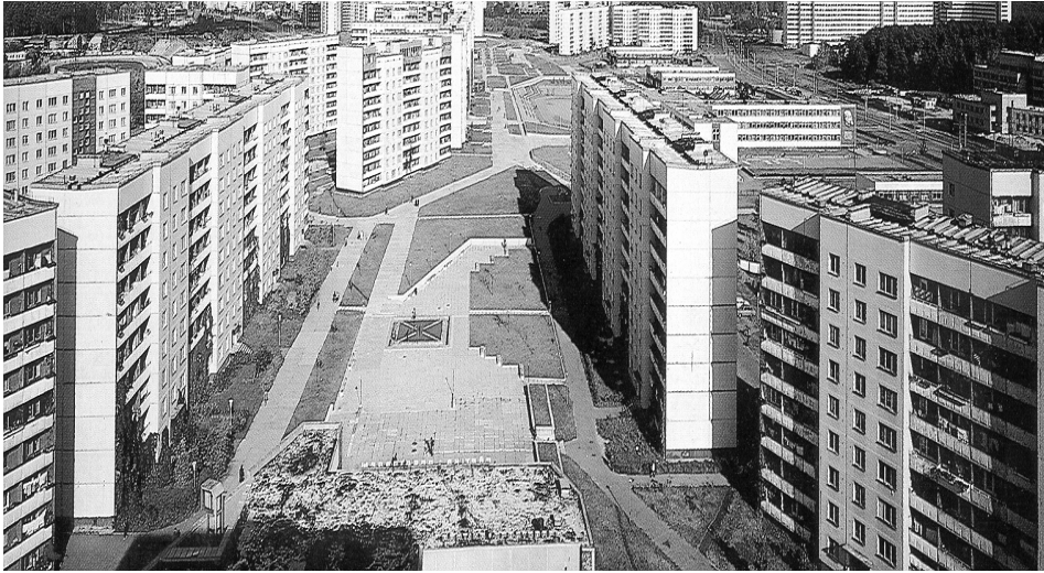
Figure 1 Mezciems, main street; nine-storey slab blocks with concrete panel façades, deteriorating retaining walls.
