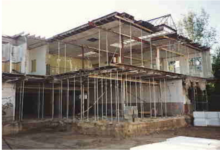
Fig. 1 A fully stripped building for re-use
