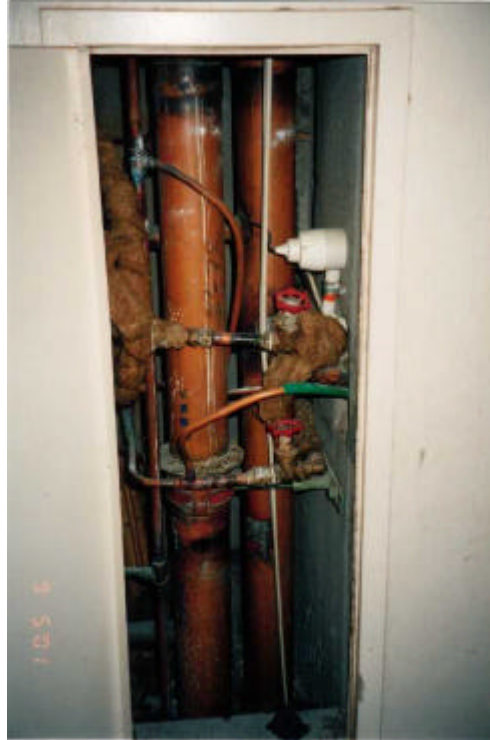
Figure 3. Access to sewer stack was an important consideration
