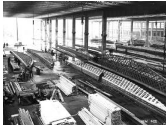
Figure 6. Fabrication of Belfast trusses c1917 (© UFTM no.426)
