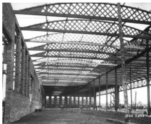
Figure 2. Aeroplane hangar construction Aldergrove 1918 (©UFTM no.H2451)
