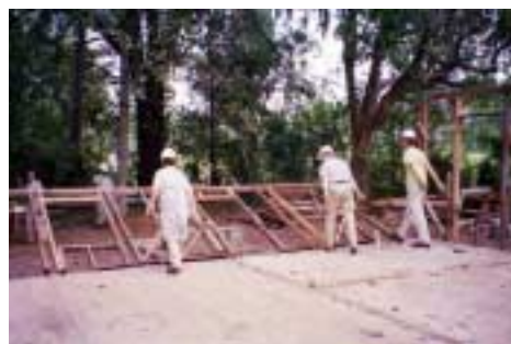
Figure 10 – Light-weight materials facilitate easy handling during deconstruction
