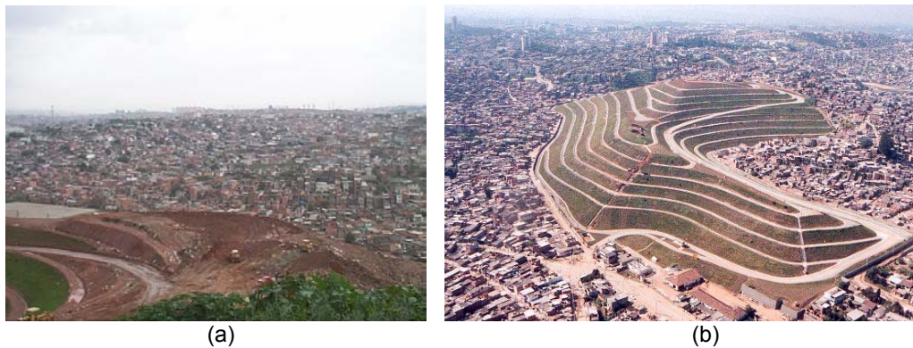
Figure 8 Itatinga, CDW class A landfill, São Paulo city. (a) during the execution and (b) after of the finalization. Source: John, V.M. and Fialho, M. A. respectively.
