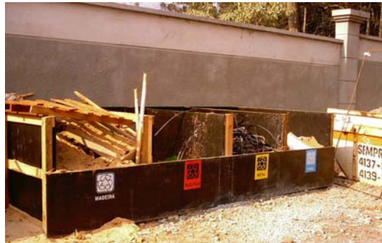
Figure 3 Selective construction waste collection in national building site. Source: Vasconcellos, F.
