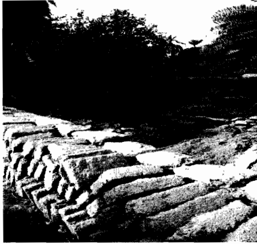
Figure 7: New adobes for a garden wall
