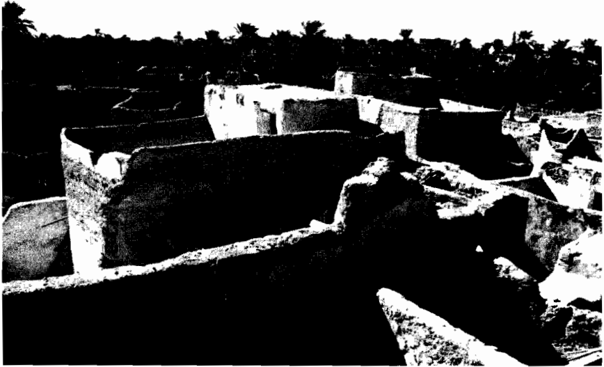
Figure 2: Detached plaster; damaged adobe substrate
