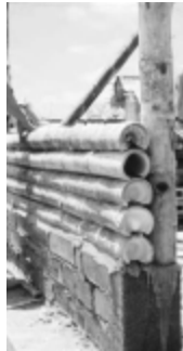
Figure 12. Walls in bamboo. Source: (Kennedy, ____:p.201)
