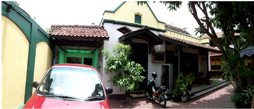
Figure 1.6 The picture of Javanese house showing the front yard and pendhapa (As batik showroom)
