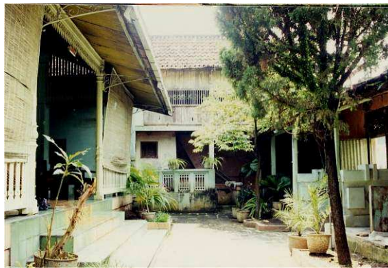
Figure 1.10 The picture of Javanese house showing the front yard and pendhapa which is now covered with bamboo curtain.
