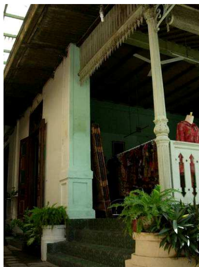
Figure 1.11 The picture of Javanese house sample B showing the main space or living room ( dalem )
